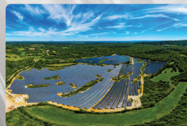
Picarreau solar farm © Corsica Sole
